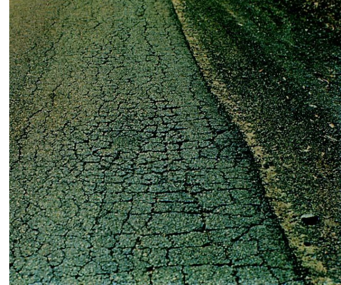
Fatigue cracking
