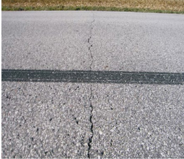
Low temperature cracking
