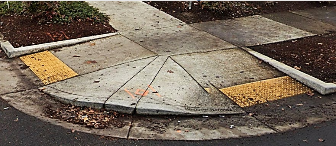
Effects of a point load (from vehicles running over concrete)
